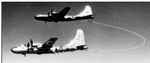
Two Boeing B-29 Superfortresses are seen here using an early air-to-air refuelling technique that was eventually superseded by later flying boom and / or probe & drogue techniques. - USAF Photo
